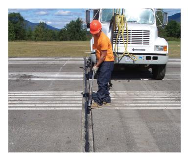
The Hot Air Lance is used to dry and prepare pavement cracks, potholes and distressed pavement surface for repair. Featuring separate valves which control the mixture of fuel and compressed air at the point of combustion.
