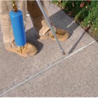
Crack-Stix<sup>®</sup> are furnished as a gray solid "rope" in 1/2" or 1/4" thickness. It is an elastomeric, self-leveling sealant, which liquefies quickly and can be used in concrete joints and cracks or faded asphalt. When properly applied, it combines tenacious adhesive power with extraordinary resiliency to protect against the infiltration of moisture or incompressibles through repeated thermal cycles of expansion and contraction.
