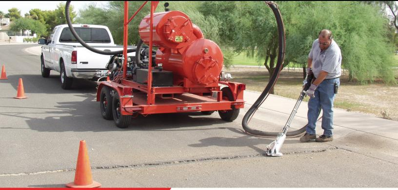
**Cleans while containing dust** and debris from the crack cleaning operation
