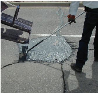
Pothole Repair
