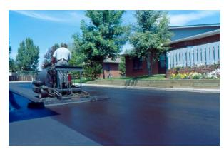
PAVISEAL seals and protects the asphalt pavement
