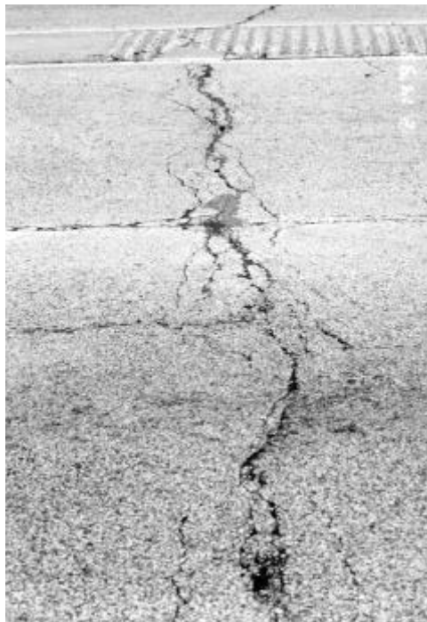
Figure 3. Pavement candidate for crack repair.
