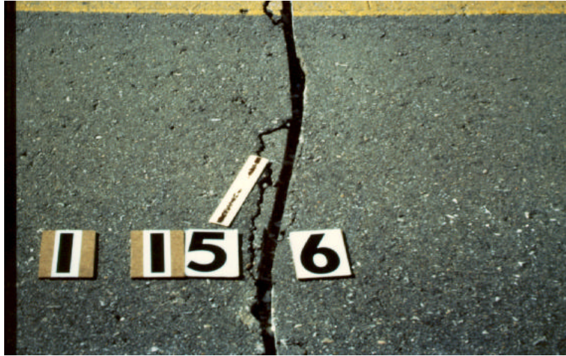
Figure 17. Crack segment missed by cutting equipment.
