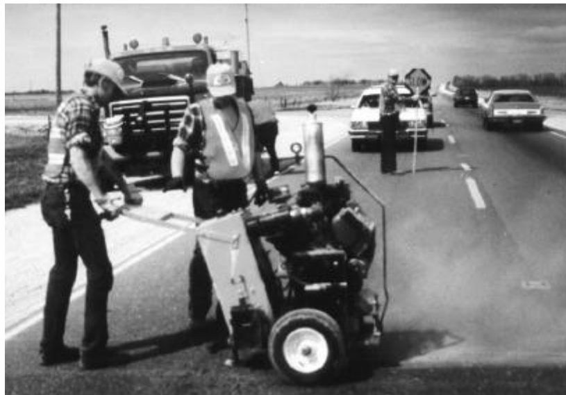
Figure 8. Diamond-blade crack saw.
