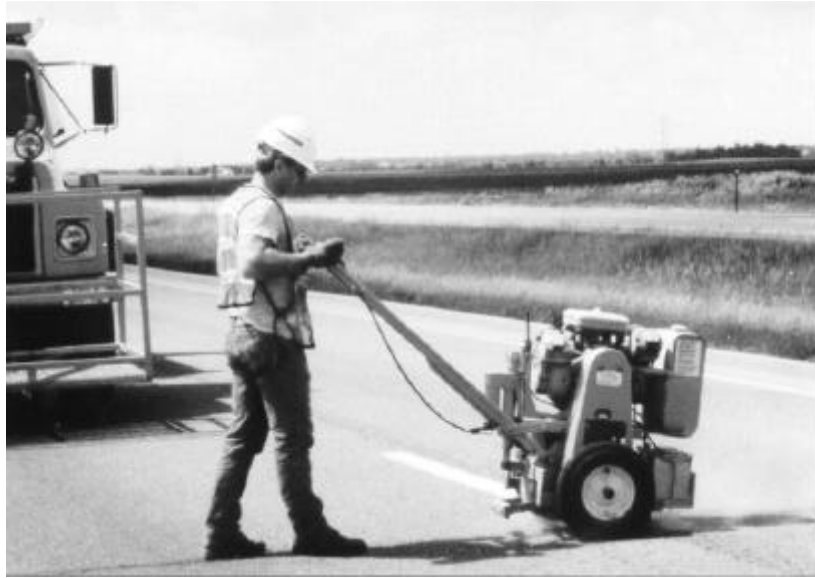
Figure 7. Rotary-impact router.
