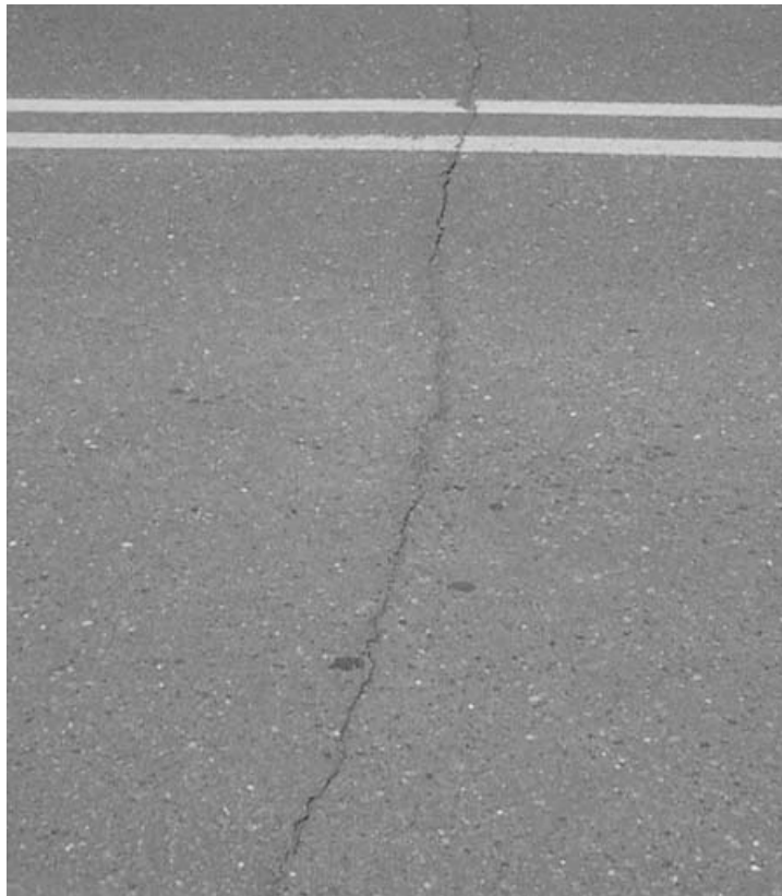
Figure 2.2 - Example of cracking with low edge deterioration
