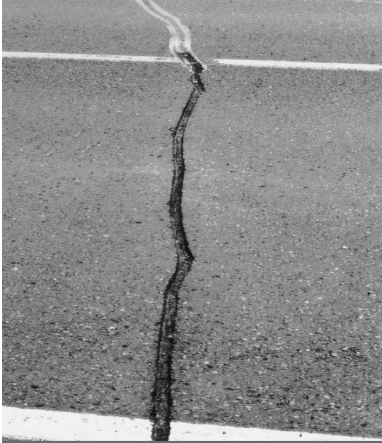
Figure 3.5 - Properly cut crack
