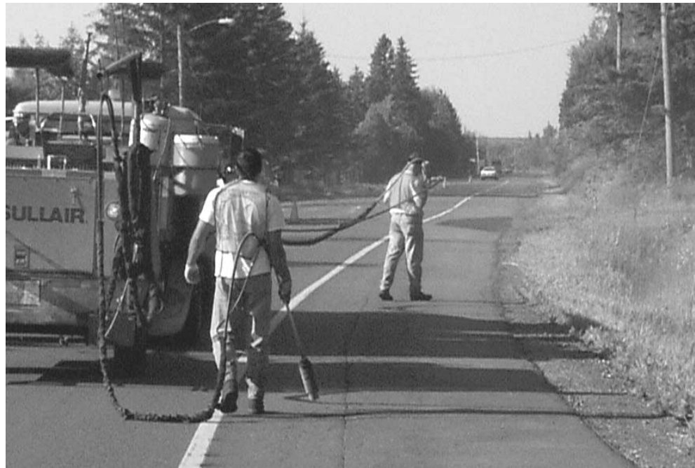
Figure 3.7 - Crack cleaning through high-pressure airblasting followed by hot airblasting
