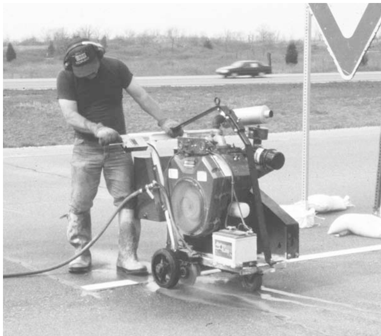
Figure 3.4 - Example of diamond saw
