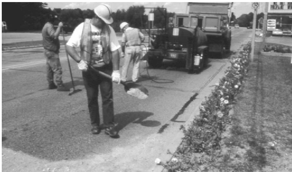
Figure 3.14 - Installation of sand as blotting material
