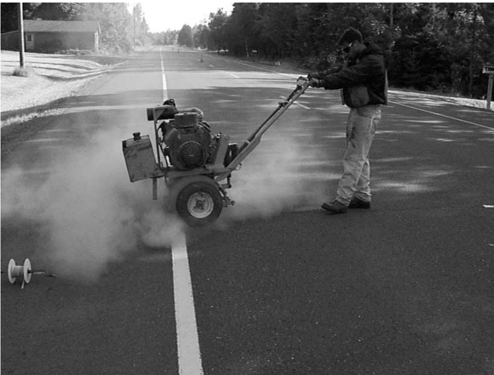
Figure 3.2 - Crack cutting using rotary impact router
