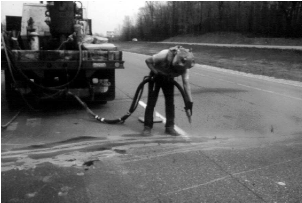
Figure 3.8 - Crack cleaning through sandblasting
