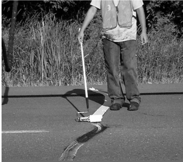
Figure 3.13 - Installation of toilet paper as blotting material
