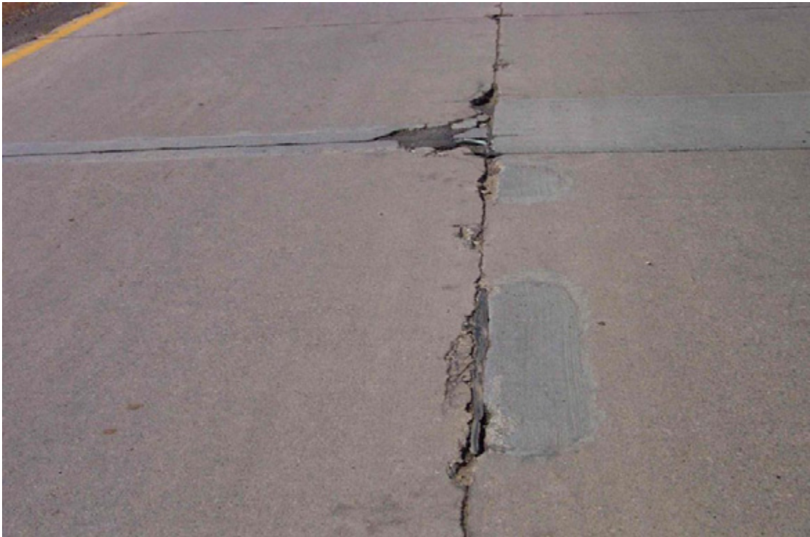
Figure 31. High Severity Longitudinal Joint Spalling
