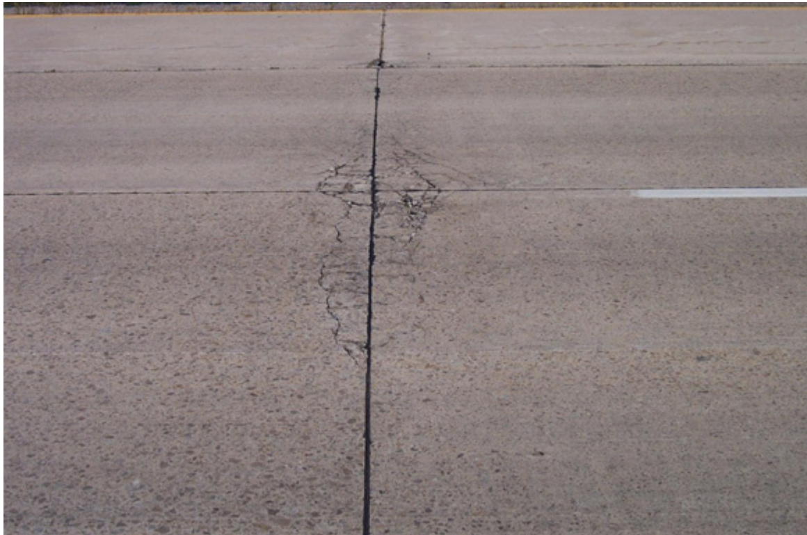
Figure 41. D-Cracking
