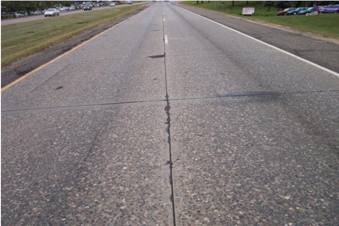
Figure 28. Low Severity Longitudinal Joint Spalling
