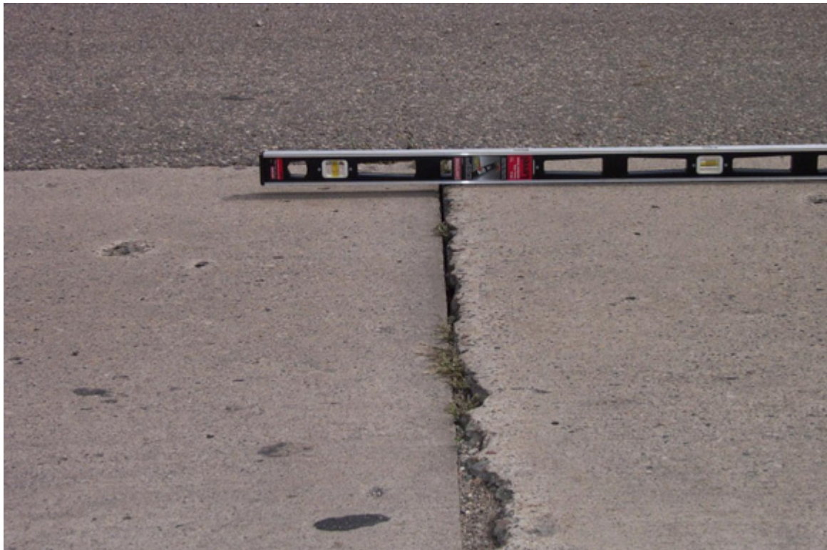
Figure 32. Faulted Joint
