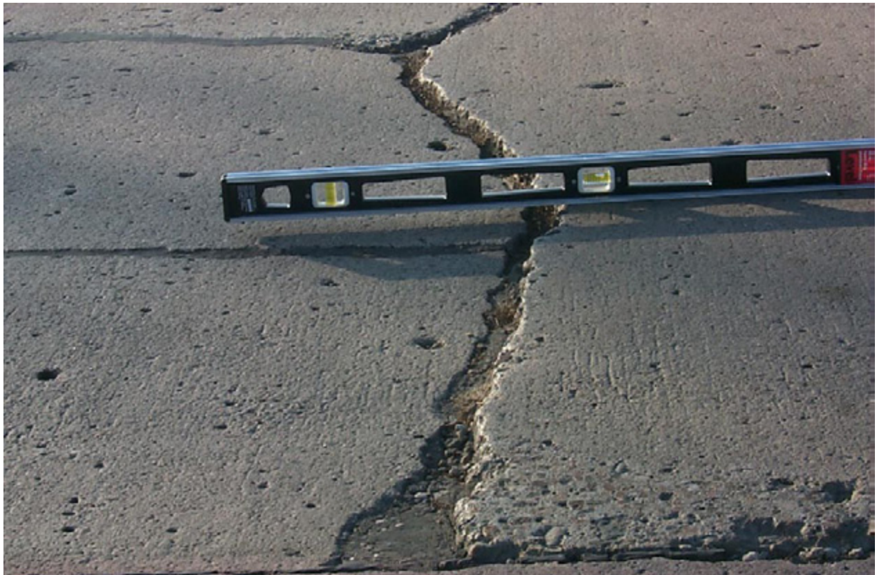
Figure 37. Faulted Panel
