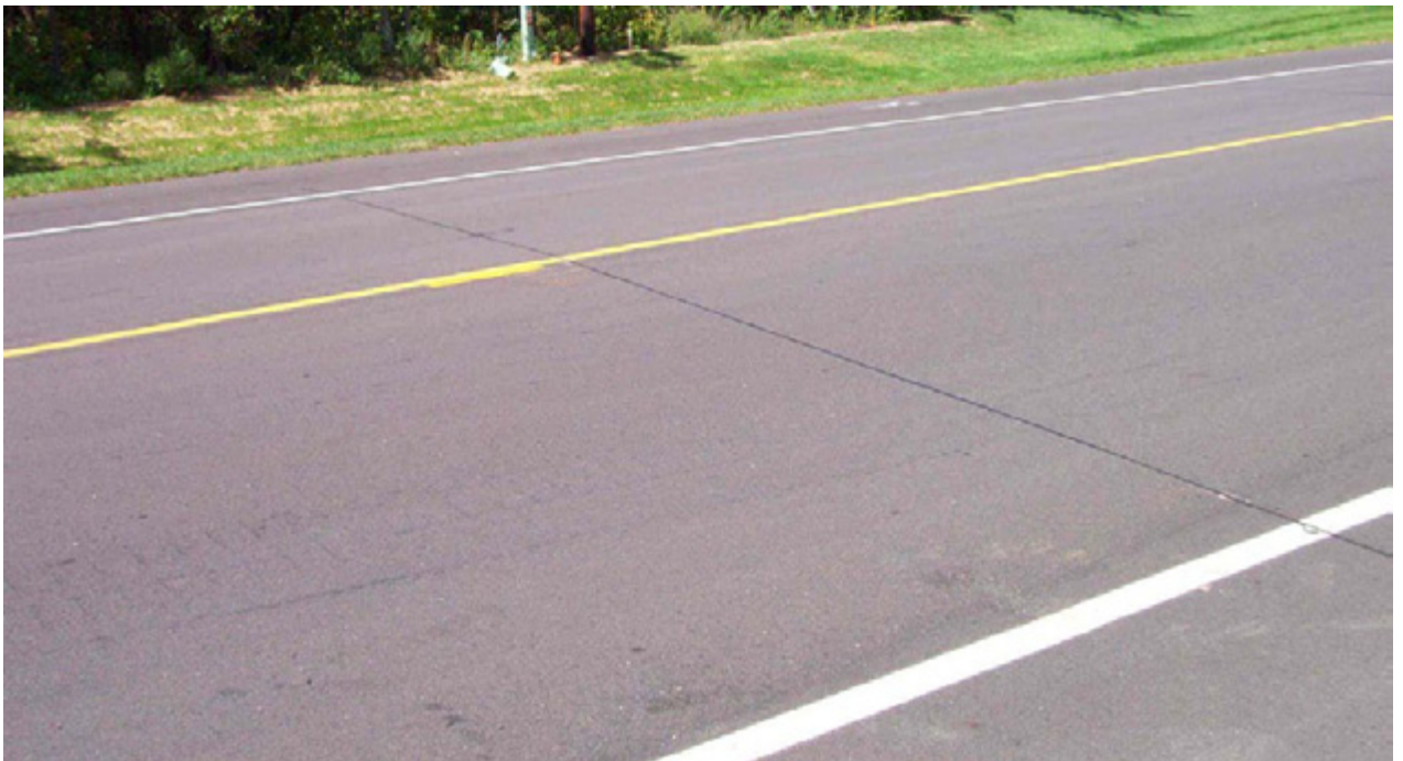
Figure 3. Low Severity Transverse - Saw and Seal
