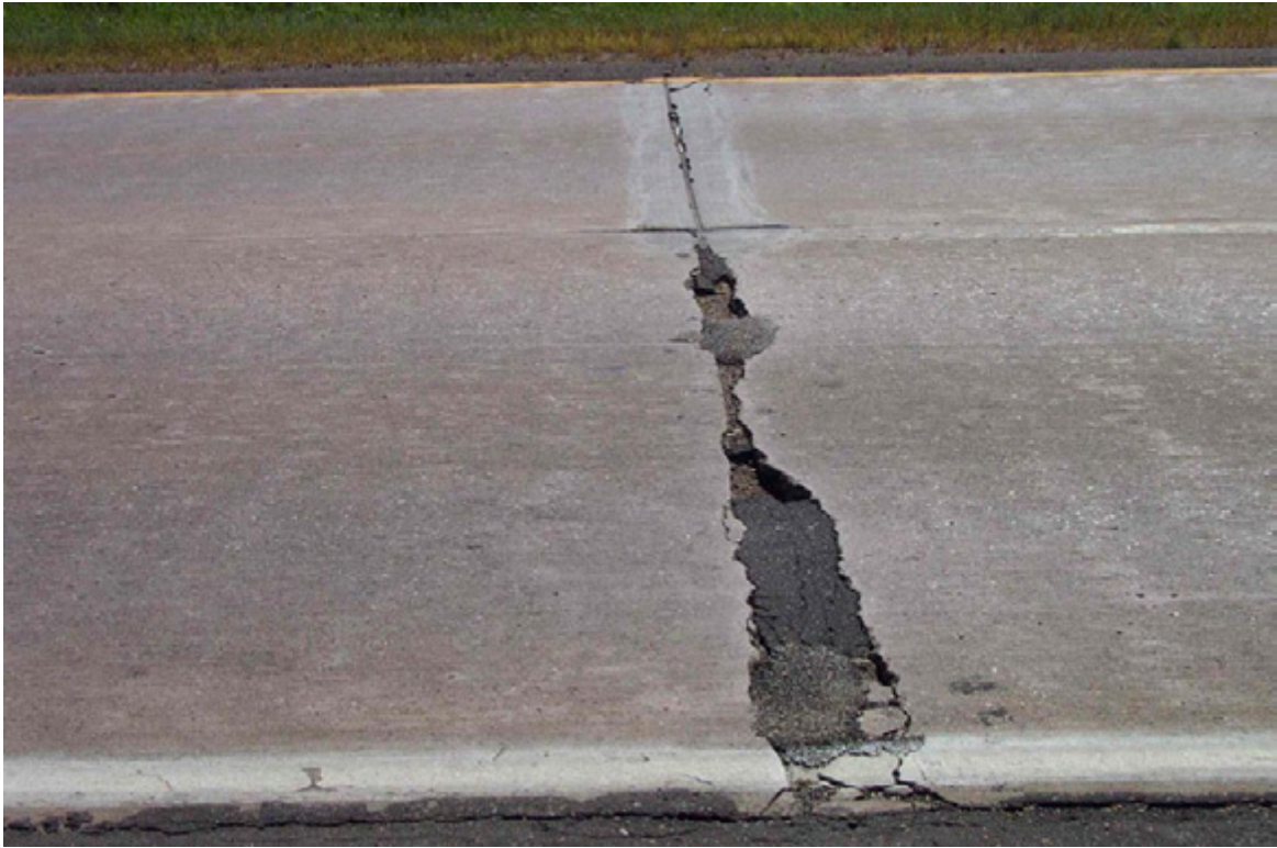
Figure 30. High Severity Transverse Joint Spalling
