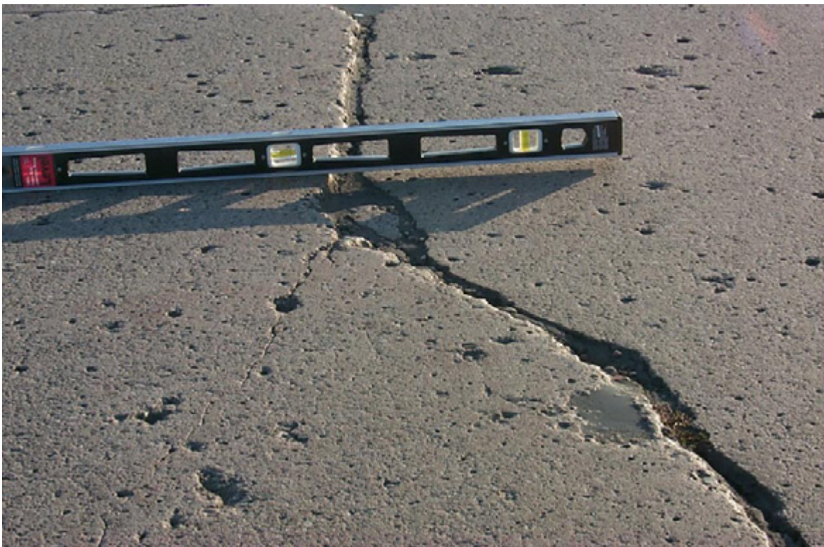
Figure 39. Faulted Panel
