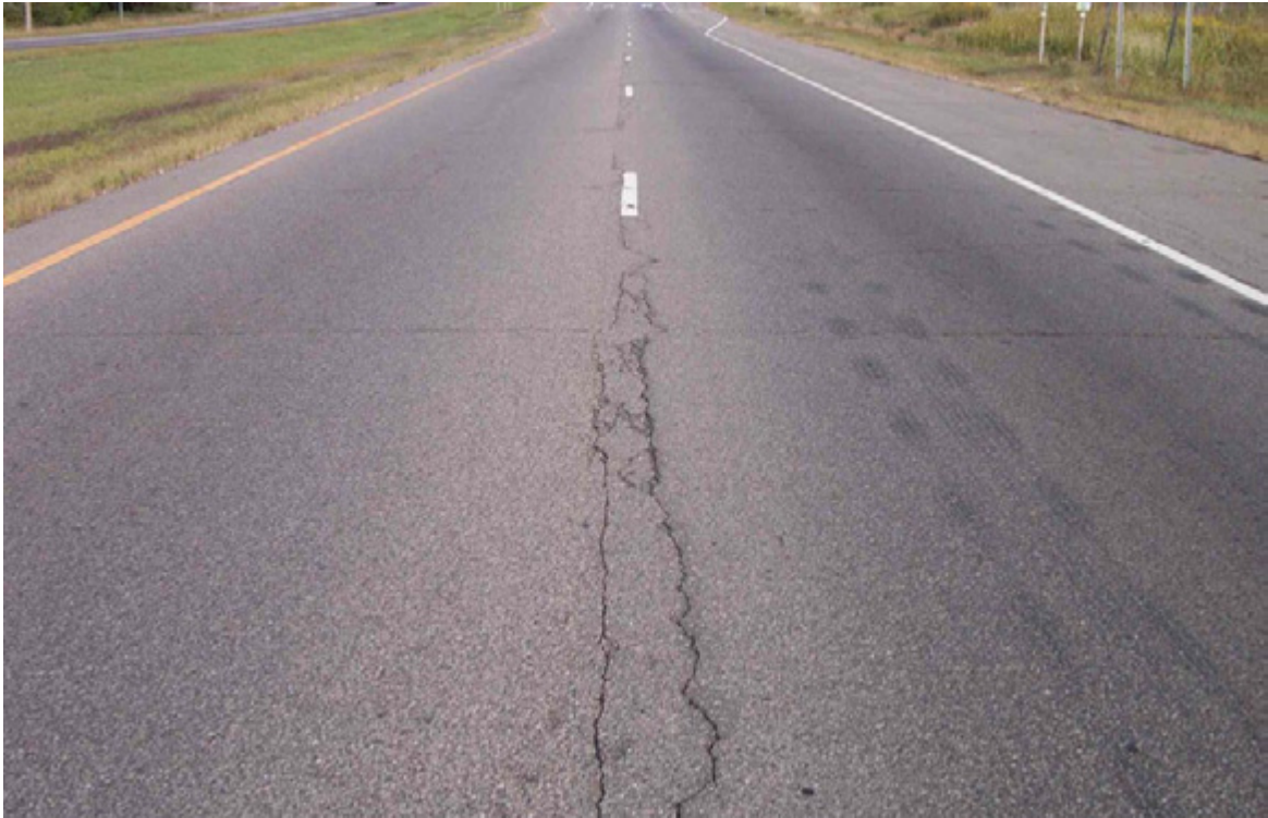
Figure 15. Medium Severity Longitudinal Joint Deterioration (random cracks)
