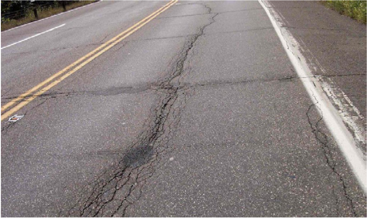
Figure 11. High Severity Longitudinal Crack (random cracks over 12" wide)
