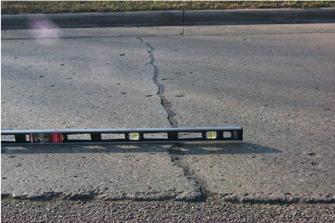
Figure 38. Faulted Panel
