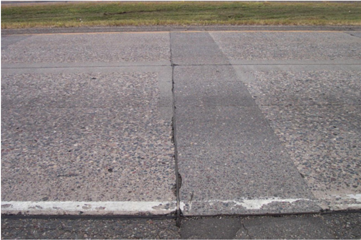
Figure 26. Low Severity Transverse Joint Spalling
