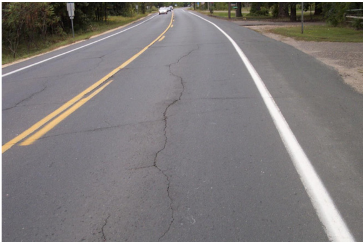
Figure 8. Low Severity Longitudinal Crack
