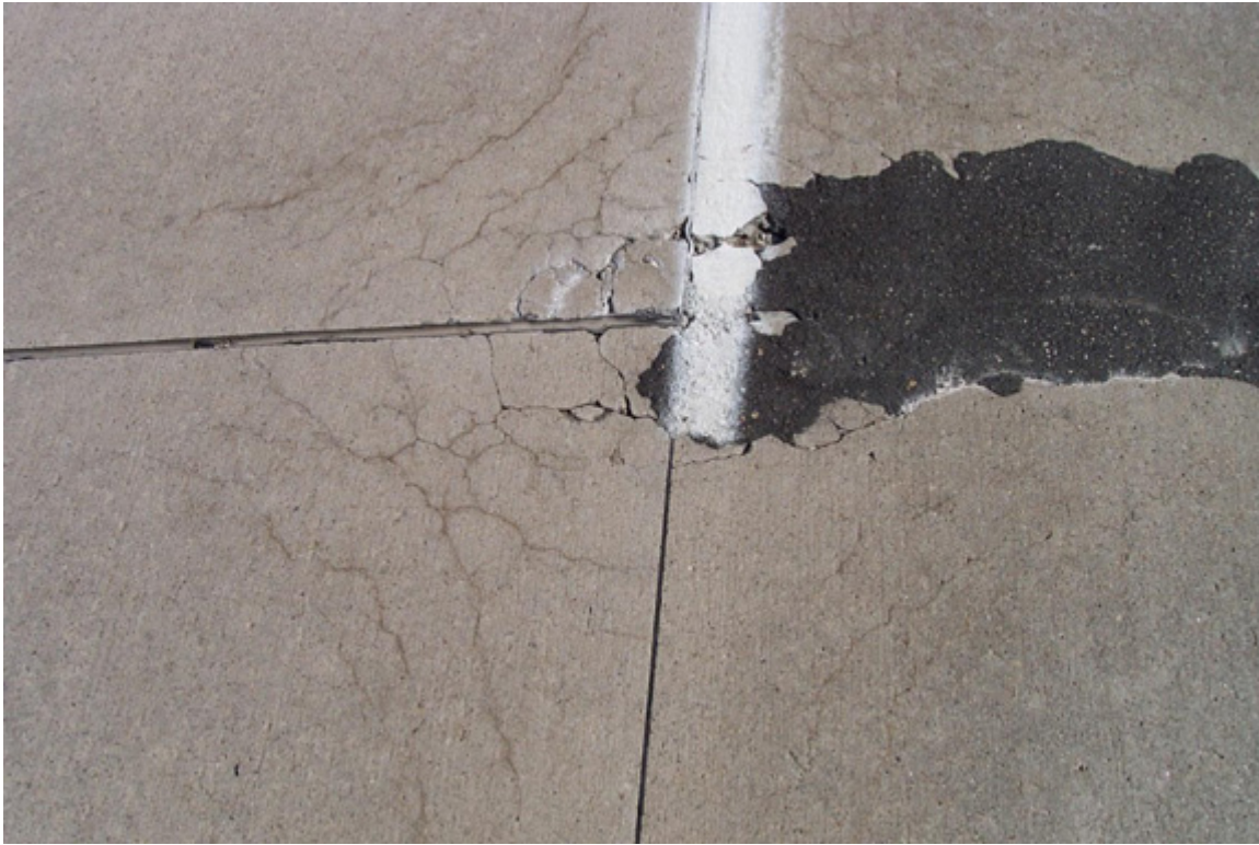
Figure 42. D-Cracking
