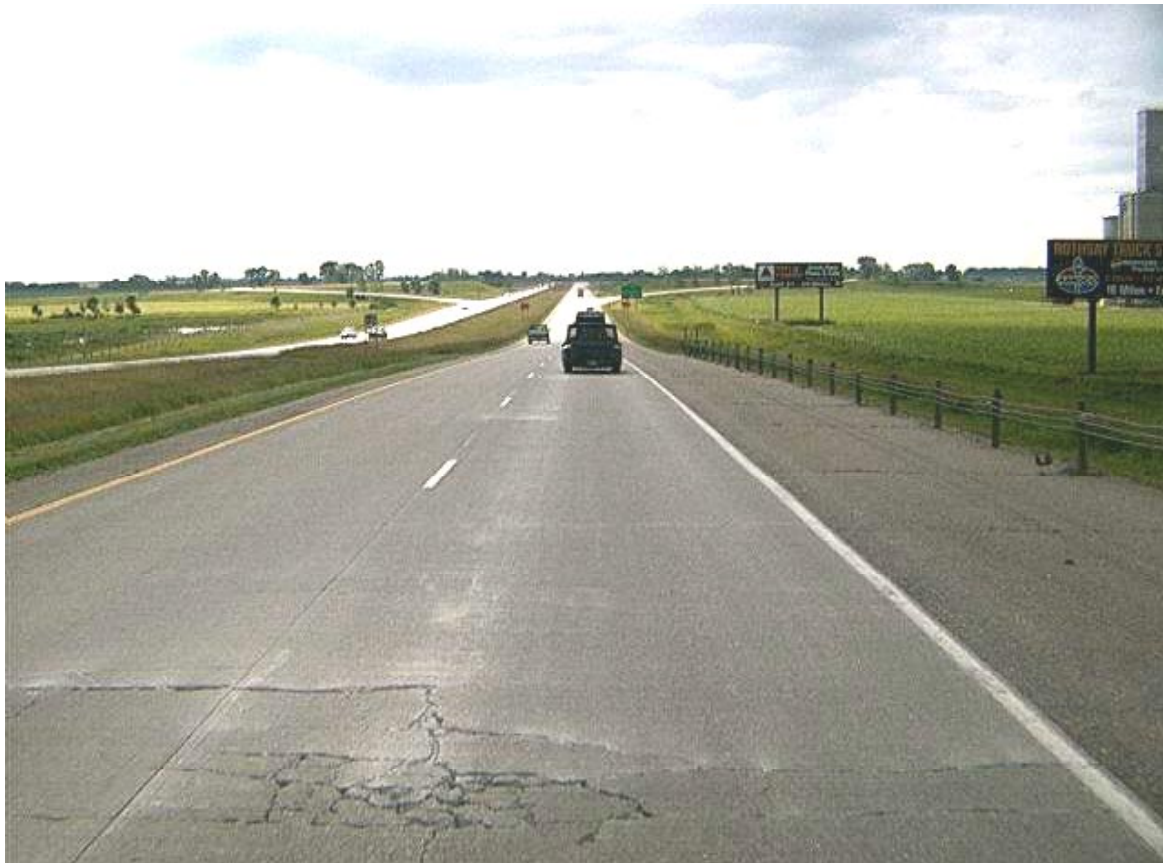
Figure 45. Localized Distress
