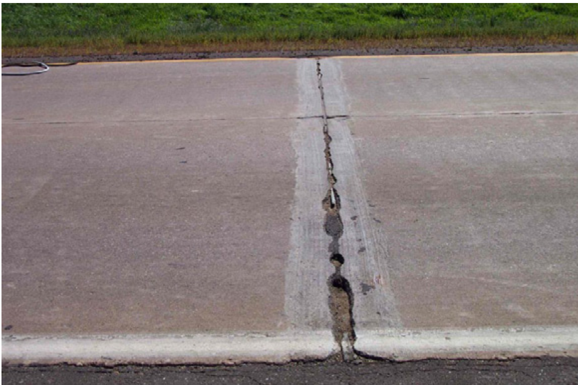
Figure 29. High Severity Transverse Joint Spalling
