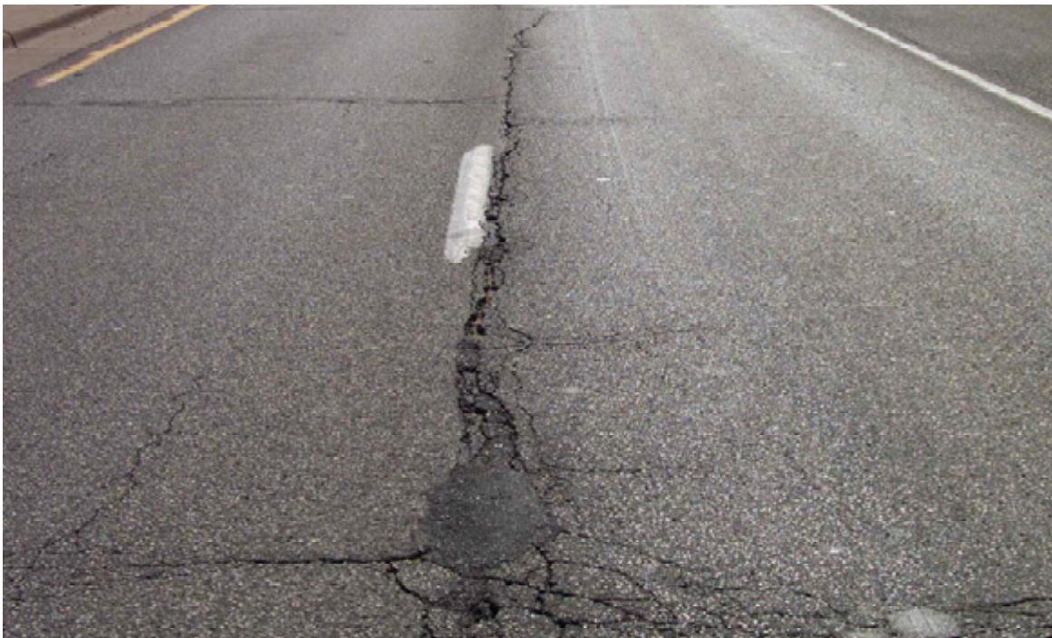
Figure 16. High Severity Longitudinal Joint Deterioration (spalling)
