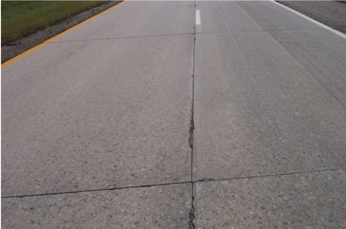
Figure 27. Low Severity Longitudinal Joint Spalling
