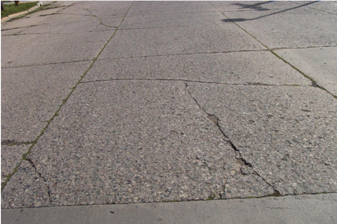
Figure 35. Cracked and Broken Panel
