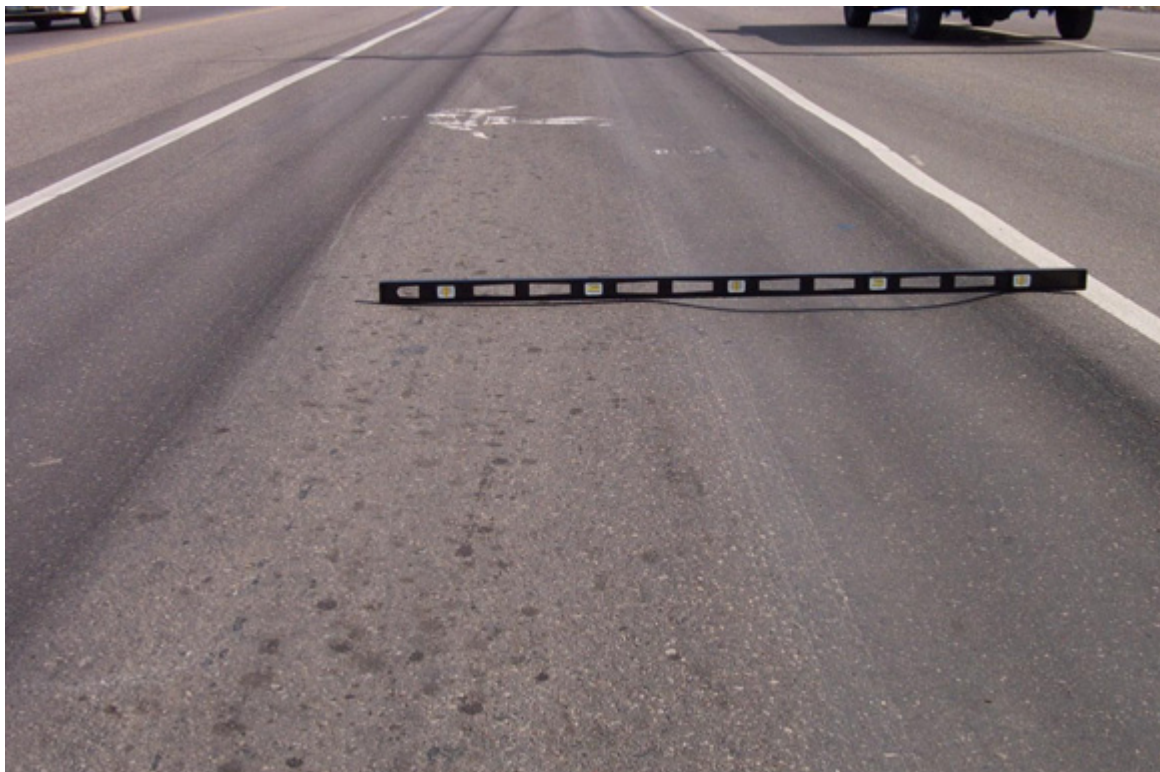
Figure 22. Rutting (0.50 inches or greater)
