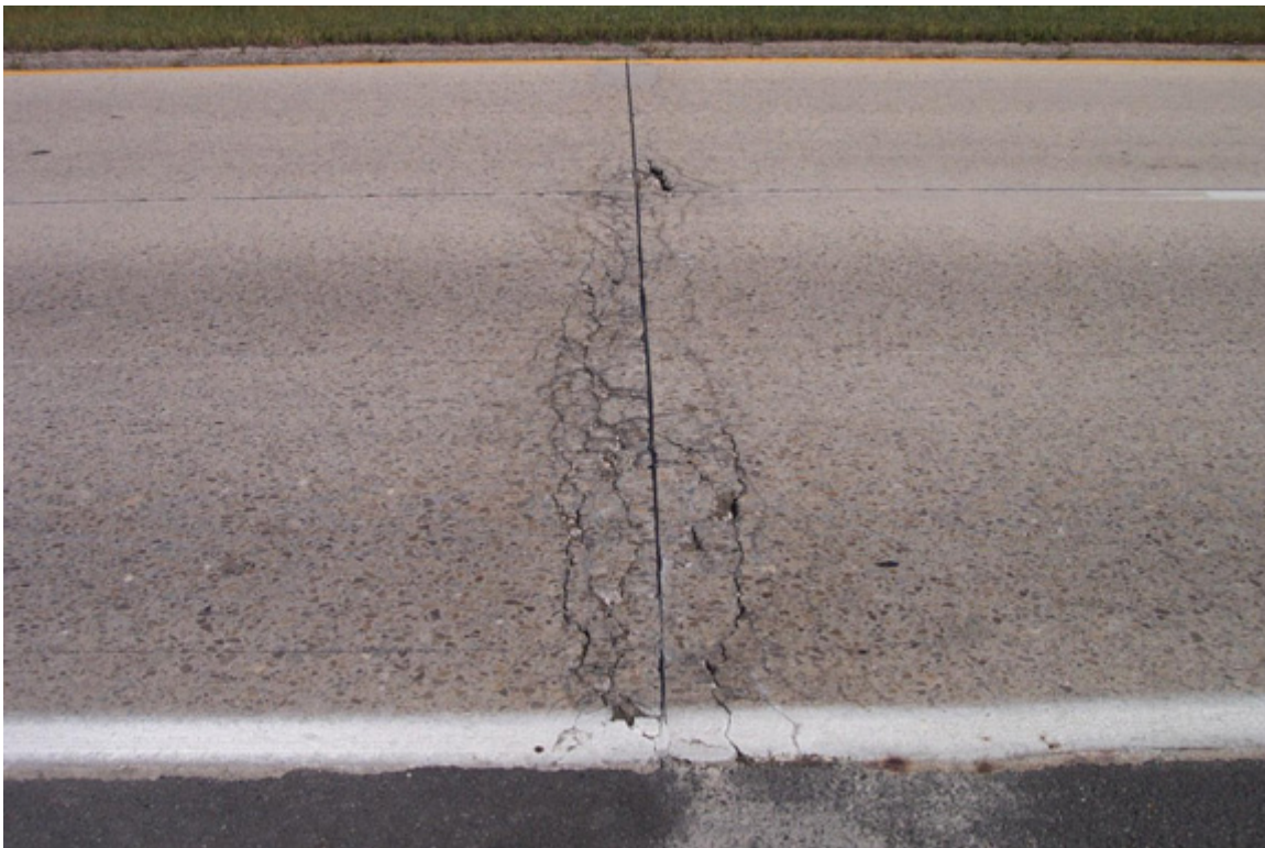
Figure 43. D-Cracking
