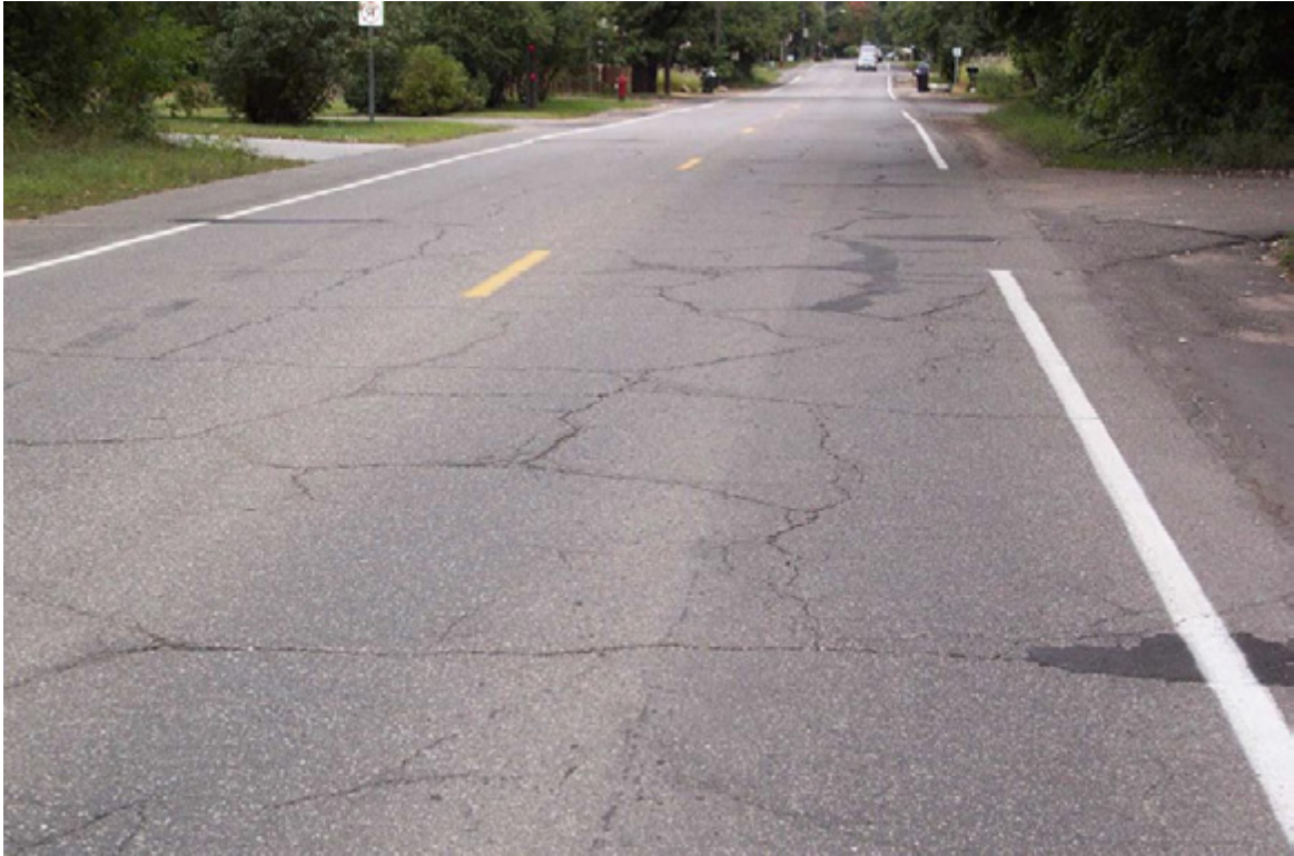
Figure 18. Multiple Cracking
