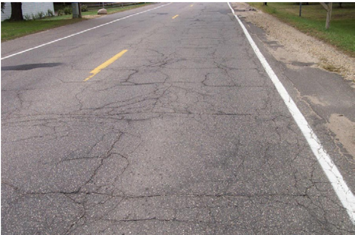
Figure 19. Multiple Cracking
