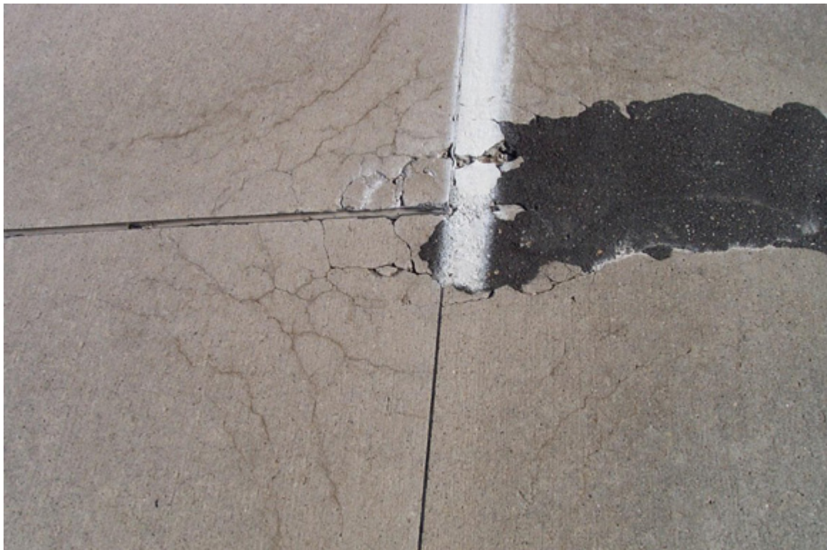
Figure 46. D-Cracking
