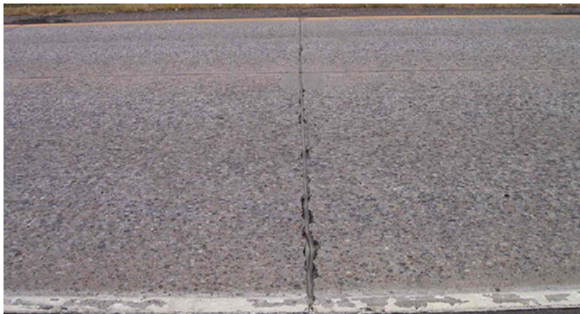
Figure 25. Low Severity Transverse Joint Spalling
