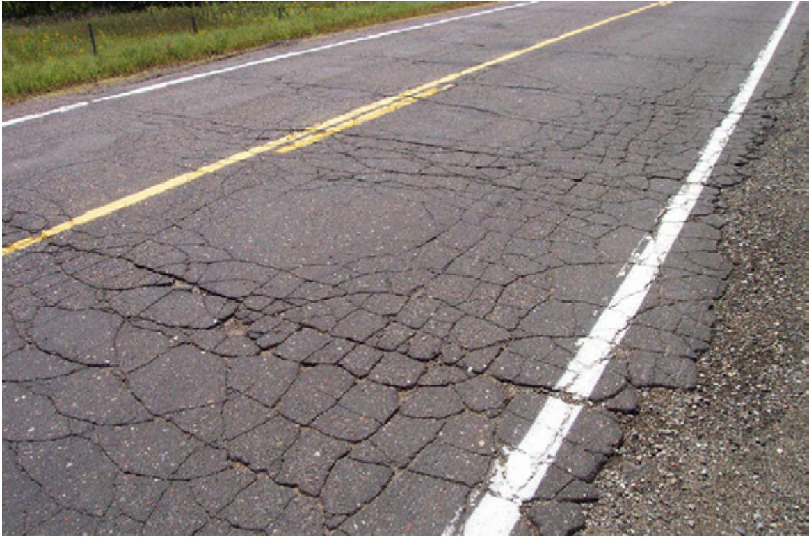
Figure 21. Alligator Cracking
