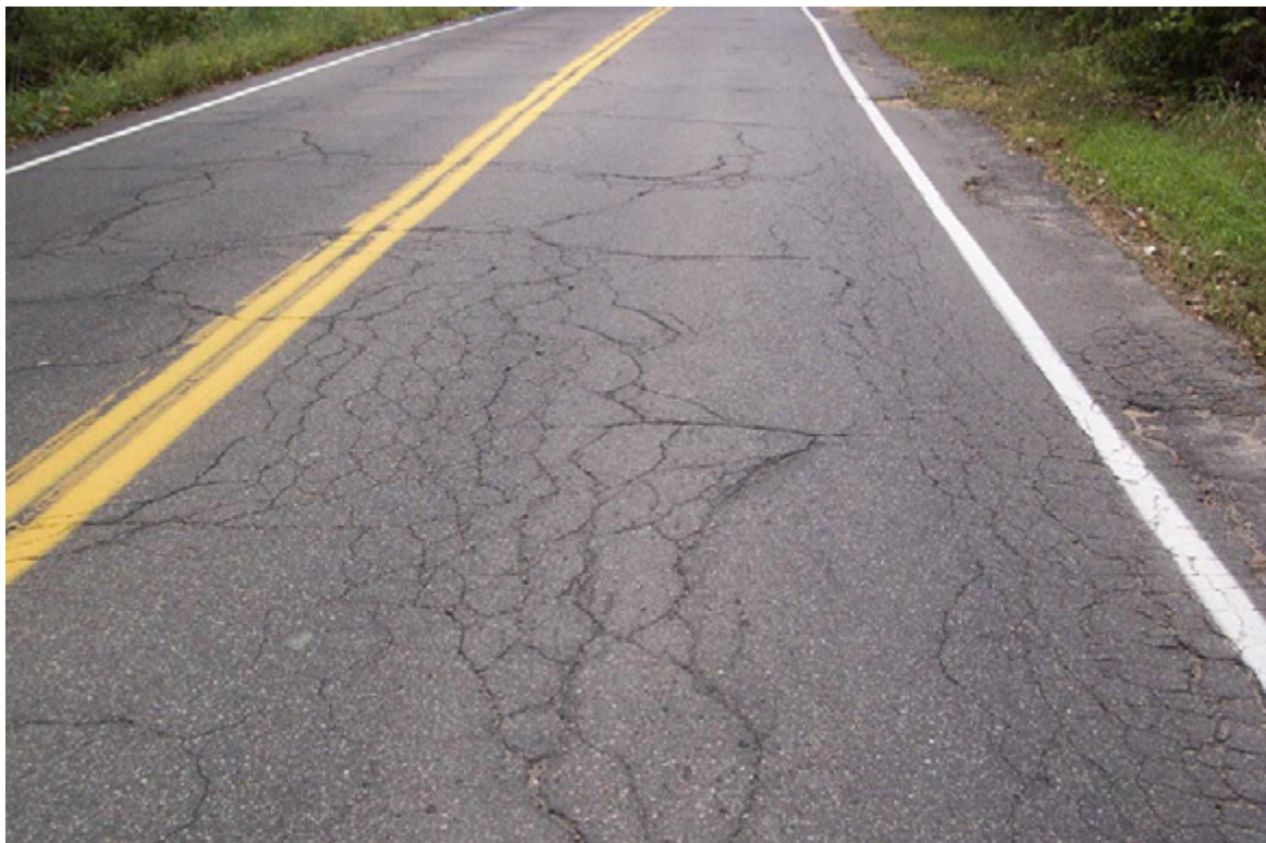
Figure 20. Alligator Cracking
