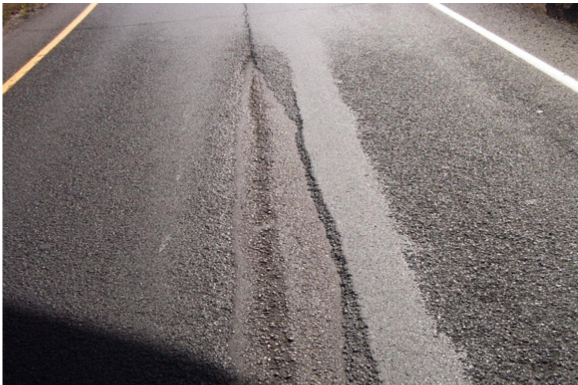
Figure 23. Raveling Under a Bridge
