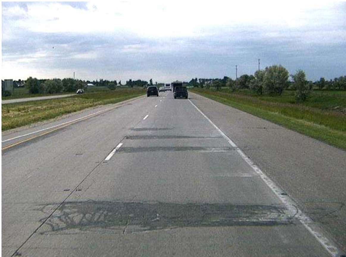
Figure 44. Patch Deterioration
