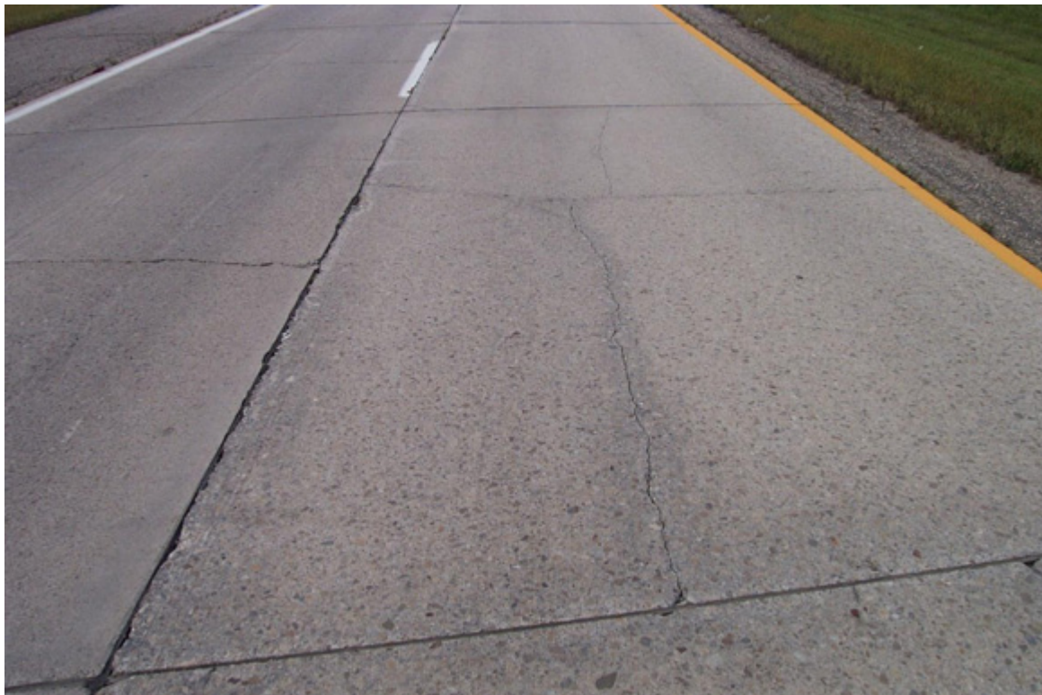
Figure 34. Cracked and Broken Panel
