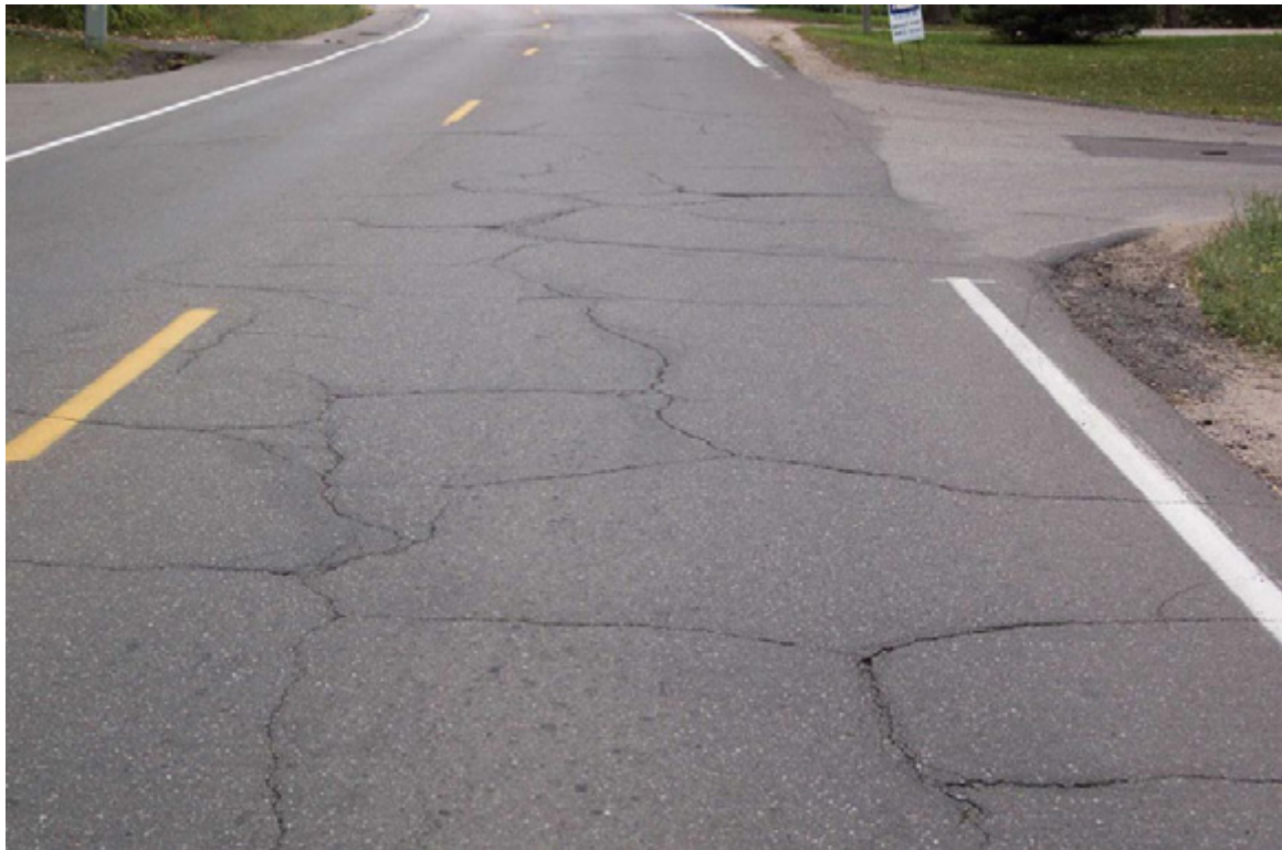
Figure 17. Multiple Cracking
