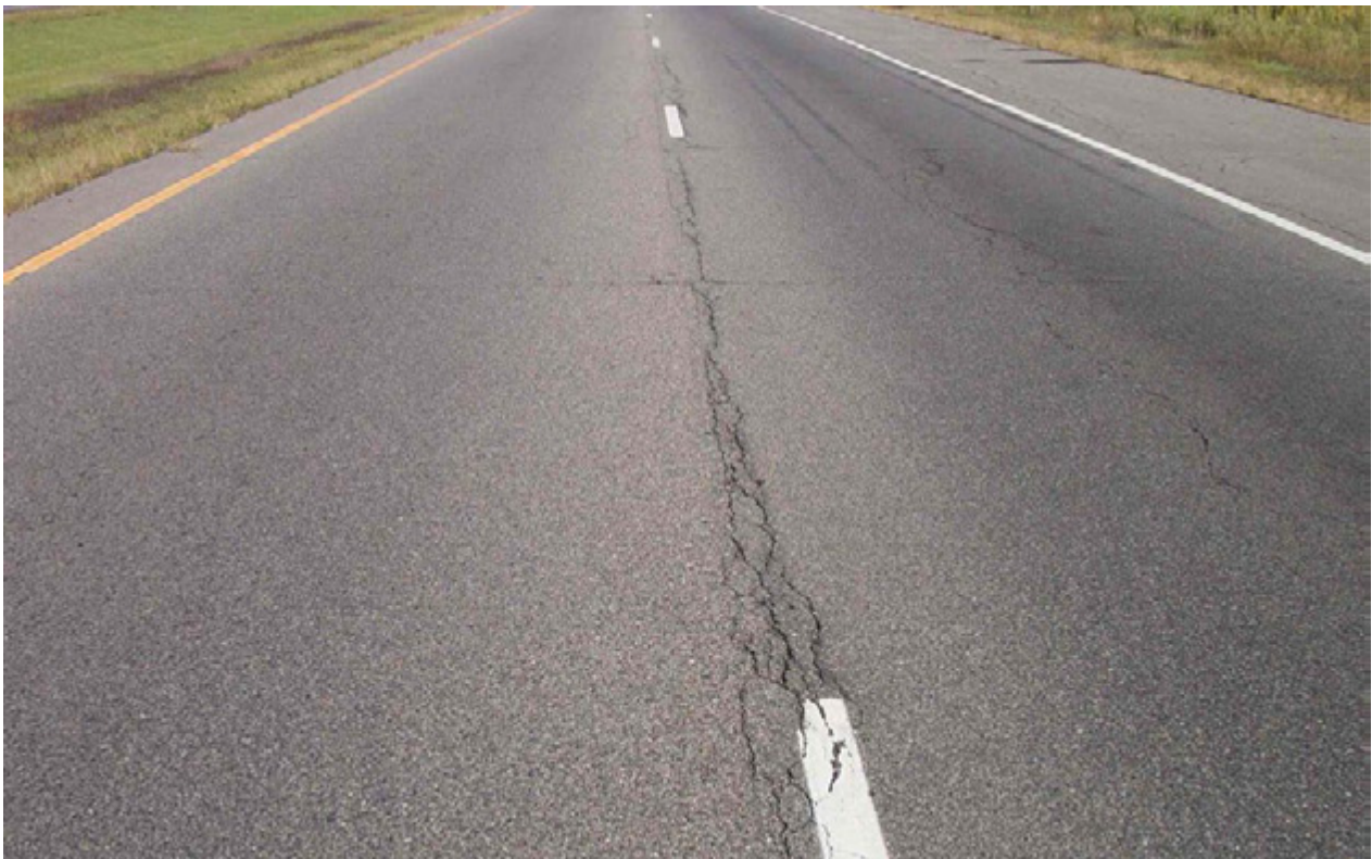
Figure 14. Medium Severity Longitudinal Joint Deterioration (random cracks)
