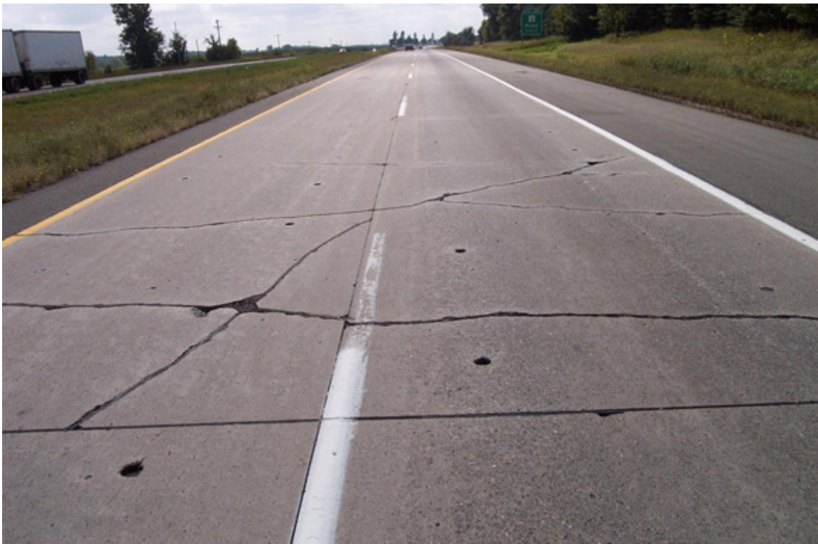
Figure 36. Cracked and Broken Panel
