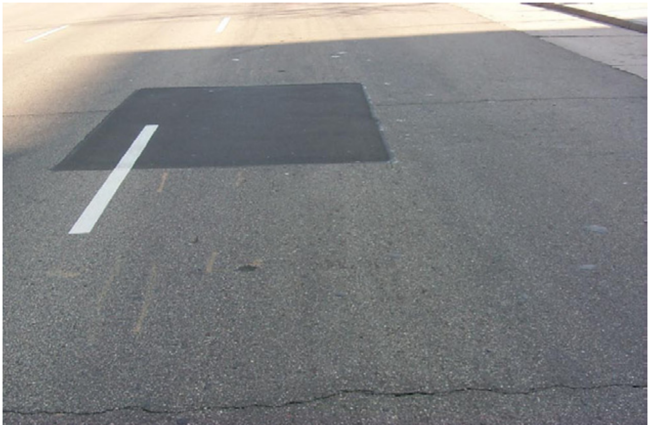
Figure 24. Bituminous Patching
