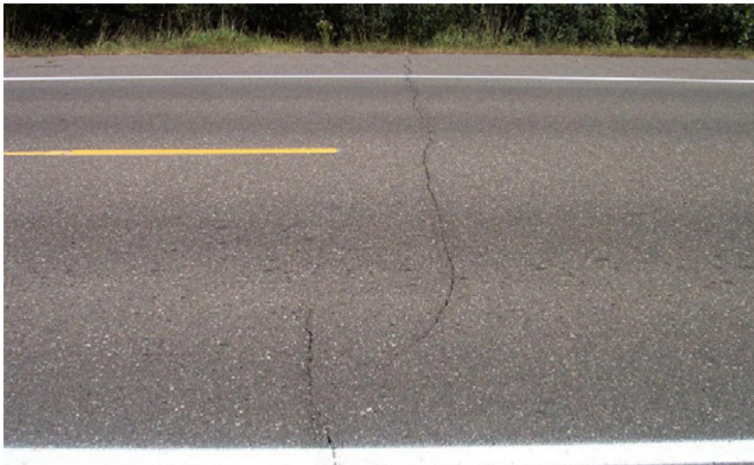
Figure 1. Low Severity Transverse Crack (no random cracks)
