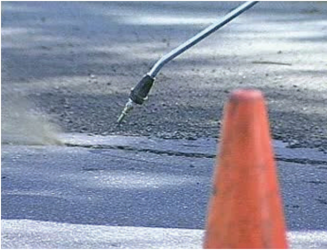
Photograph 4-7. Compressed air cleaning of crack (courtesy Crafcro).
