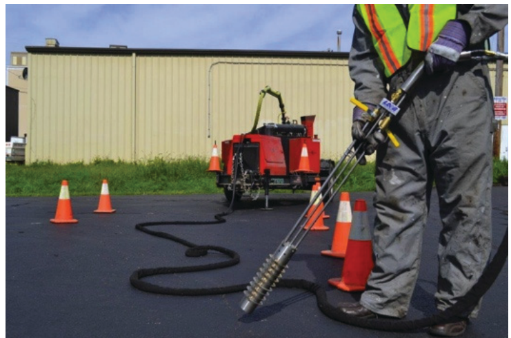
Photographs 4-9. Hot air lances (left: courtesy Crafcro, right: courtesy Lab Mfg.).
