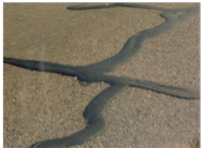
Photograph 4-3. Excessive overbanding (22).
