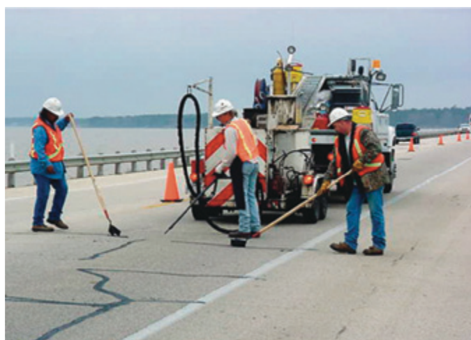
Photograph 4-15. Crack treatment operations (21).
