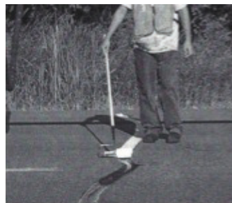
Photographs 4-14. Blotter applications: (a) Sand blotter (16), (b) Toilet paper (16), (c) Anti-tracking solution (photo by Dale Decker).
