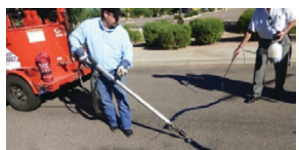
Photographs 4-14. Blotter applications: (a) Sand blotter (16), (b) Toilet paper (16), (c) Anti-tracking solution (photo by Dale Decker).
