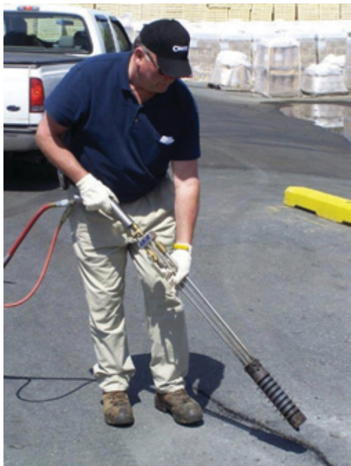
Photograph 2-4. Hot air lance (courtesy CrafcO).
