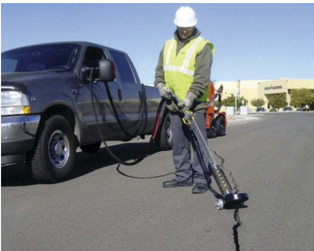
Photographs 4-9. Hot air lances (left: courtesy Crafcro, right: courtesy Lab Mfg.).
