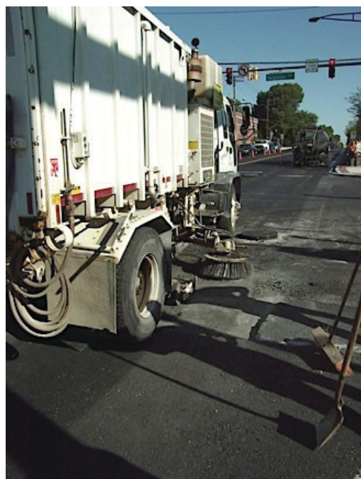
Photograph 4-6. Pavement sweeping (photo by Dale Decker).
