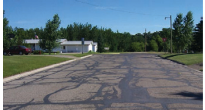
Photograph 2-2. Excessive crack filling (photo by Dale Decker).
