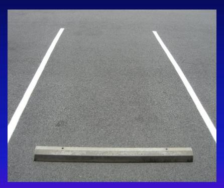
Pavement surfaces to be treated with rejuvenators should be clean and dry and free of all dirt, sediments and other debris prior to application of the product.
