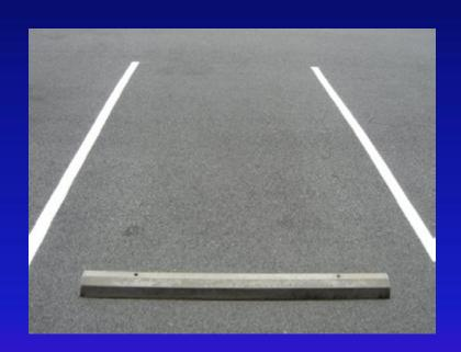
Pavement surfaces to be treated should be clean and dry and free of all dirt, sediments and other debris prior to application.
