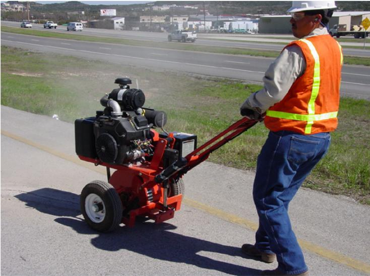
*Figure 8. Crack Routing Procedure*
